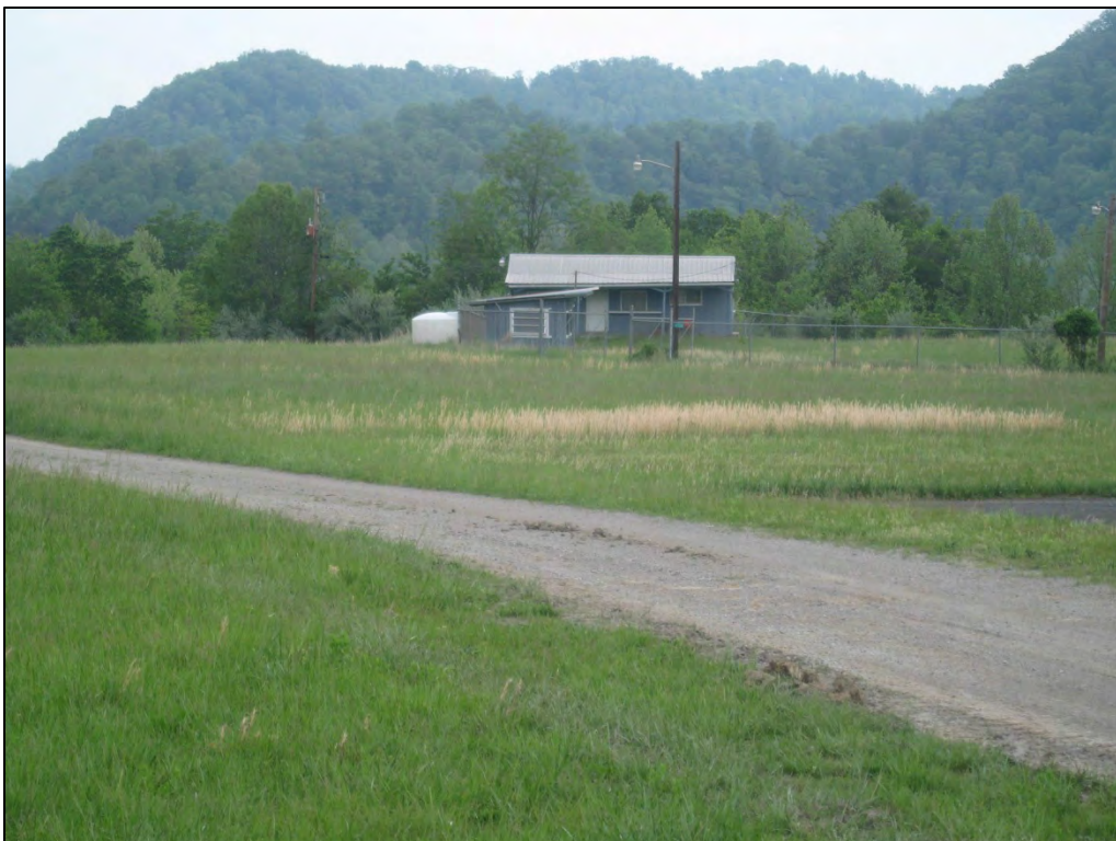
Photo #4 – Buildings on Roxana Site
