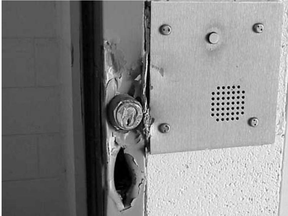
**Locking mechanism destroyed by weight bar**
