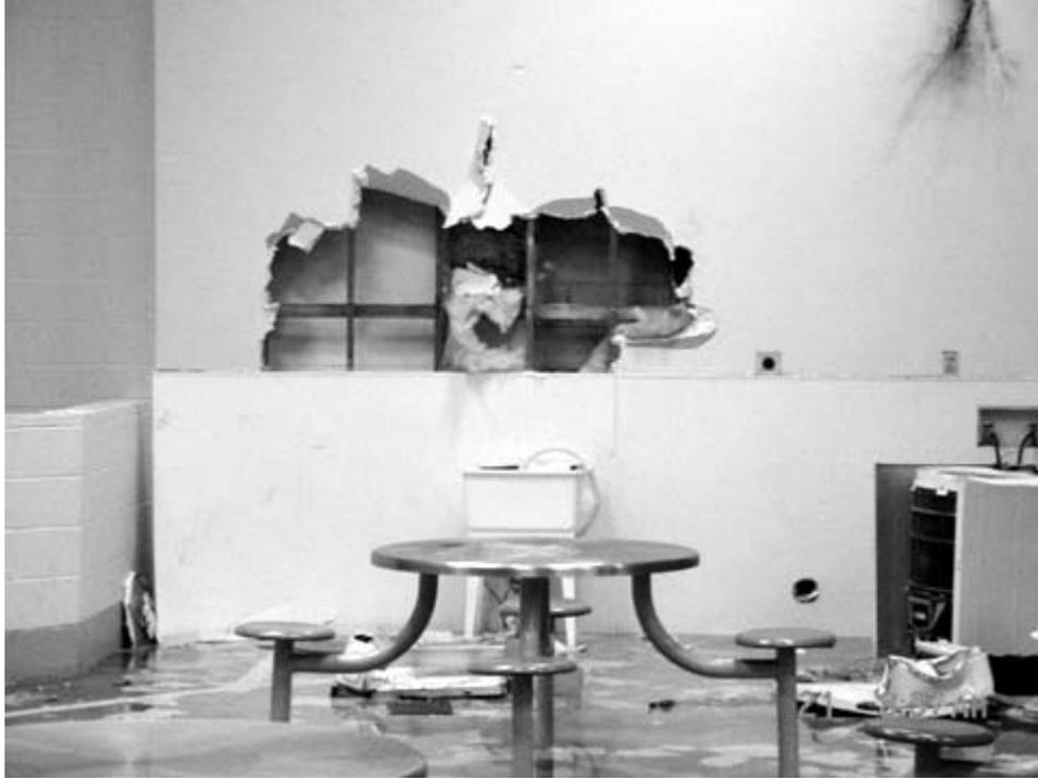
**Housing Unit: Damage to sheetrock and flooding**
