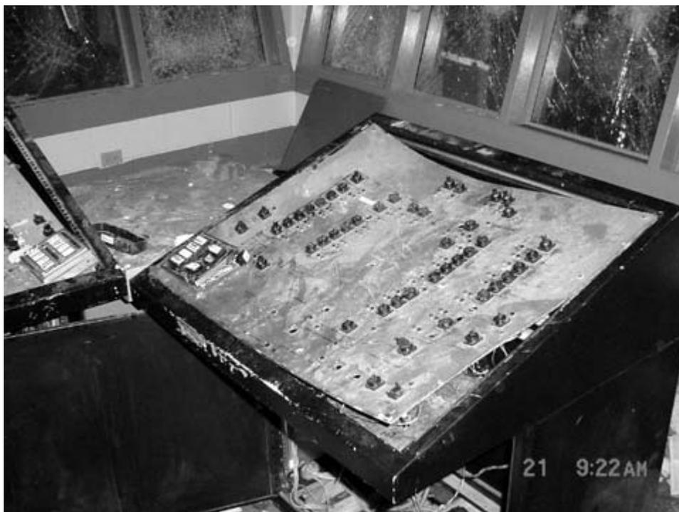
**Housing Unit Control Center: Electronic panel destroyed**
