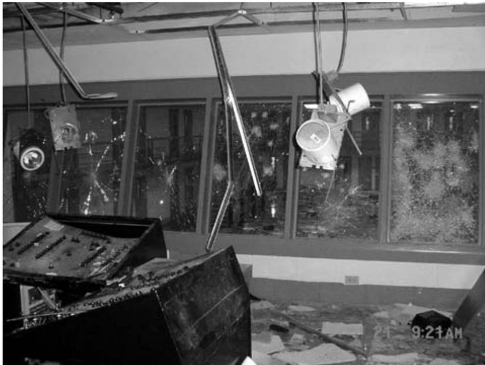
**Housing Unit Control Center: Inmates gained access and damaged sprinkler systems, control panel and windows overlooking unit.**
