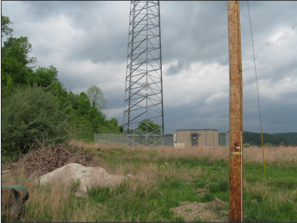
Photo #7 – Cell Tower on Van Fields Property
