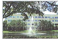
EASTERN REGIONAL OFFICE Palm Beach Gardens, FL
