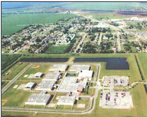
The South Bay Correctional Facility near the shores of Lake Okeechobee in central Florida
