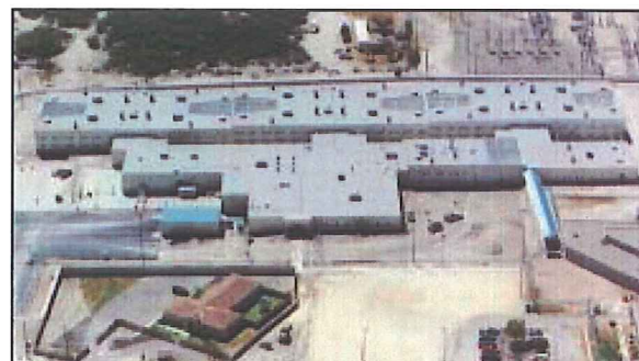
The new Val Verde Correctional Facility adjoins the renovated jail
