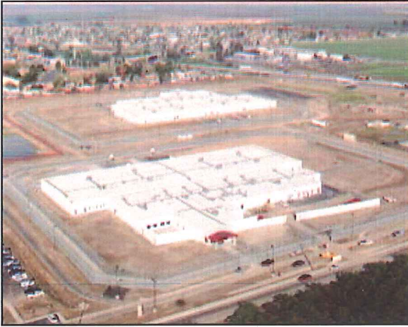
Construction finishes at Central Valley & Golden State
