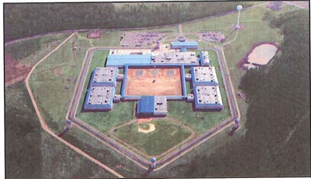
The Rivers Correctional Institution in Winton, North Carolina was completed on time and within budget for the March 2001 opening.
