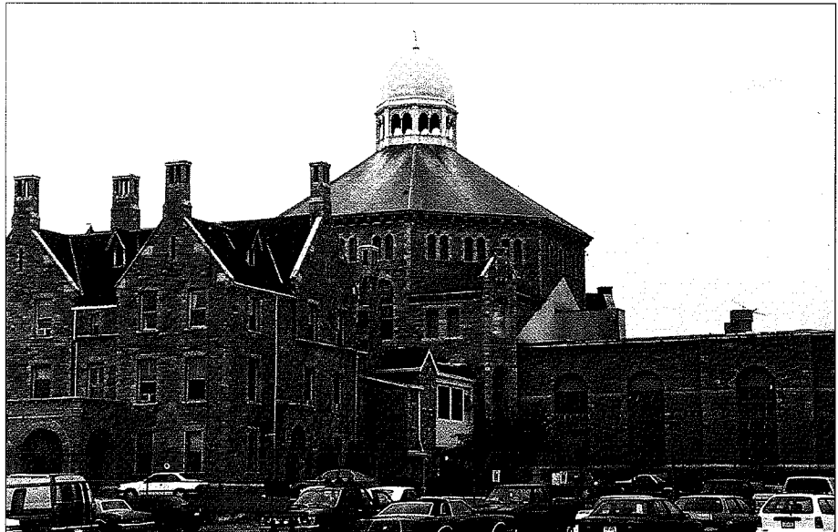
"Old Max," the building where maximum security prisoners are housed, has been extensively renovated.
