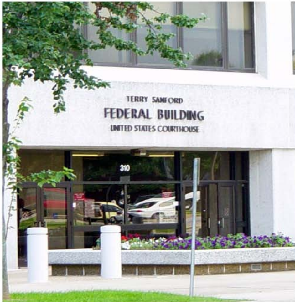
The Federal Courthouse, Raleigh, NC
