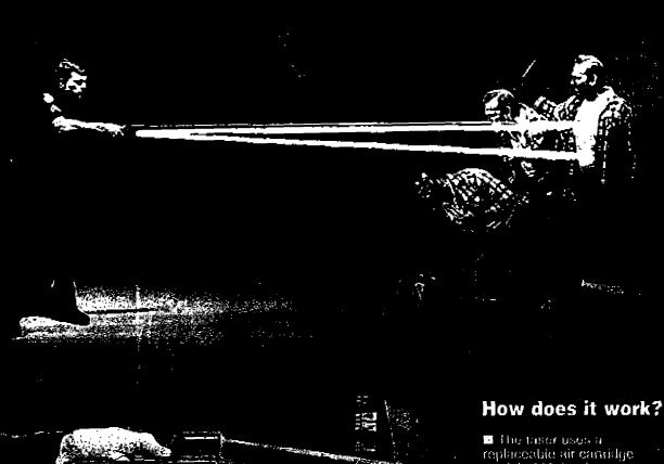
The taser uses a replaceable air carridge module (1) that fires out two probes (2) up to 15 feet at a speed of 135 feet per second. These probes are connected to the power bandle by a high-voltage insulated taser wire (3). When the probes make contact with the target. 50,000-volt impulses are carried along the taser wire and into the suspect. These taser waves (4) can penetrate 2 comulative inches of clothing, including , leather.
